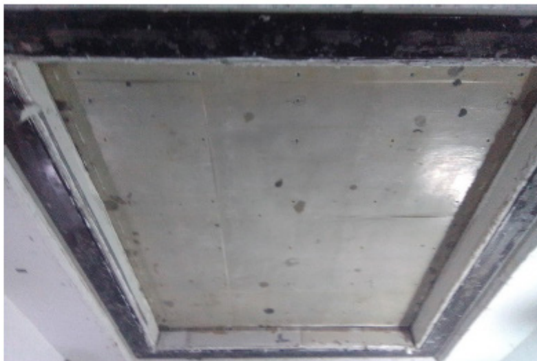
Photo No. 2 Receive Room View of Test Specimen Installation
